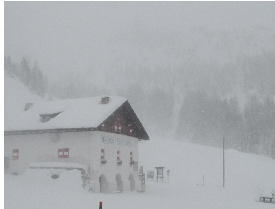
Wind, snow, and no roof make things harder (picture taken by a webcam)
